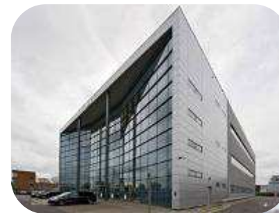
New biologics R&D centre - Slough, U.K.
