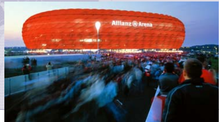
Munich football stadium, covered with ETFE plastic film.
